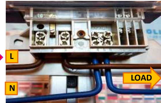
Wiring to meter terminals
