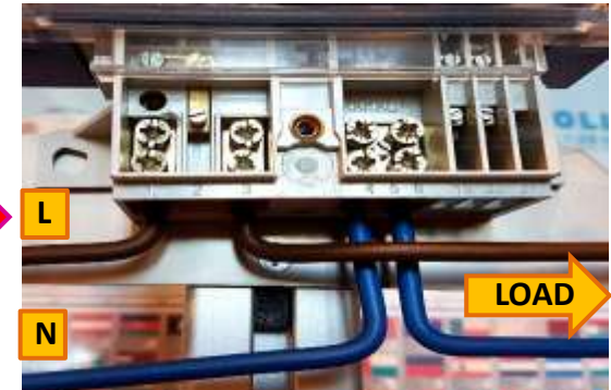
Wiring to meter terminals
