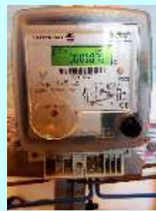
Typical single phase electronic meter with LED and its parameters
