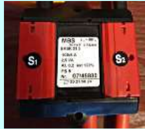
Typical current transformer CT in metering installation
