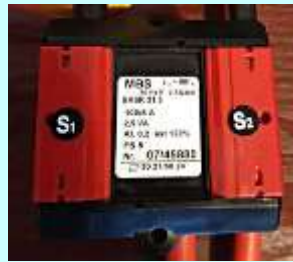
Typical current transformer CT in metering installation
